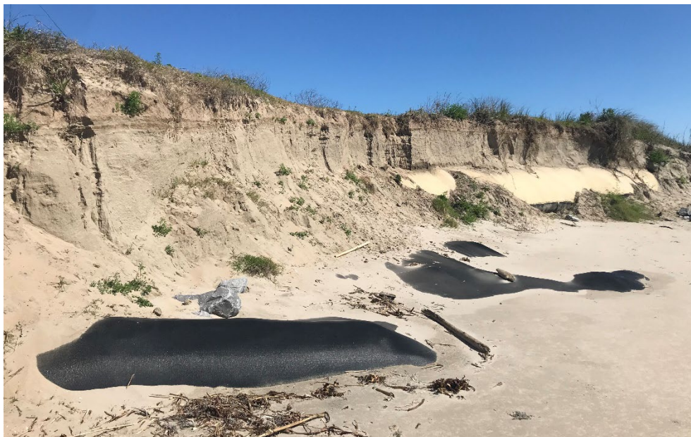
Figure 12: Exposed Geotube
