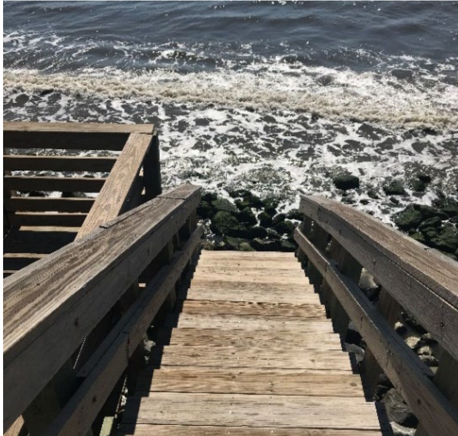
Figure 11: Boardwalk Closed Due to Erosion
